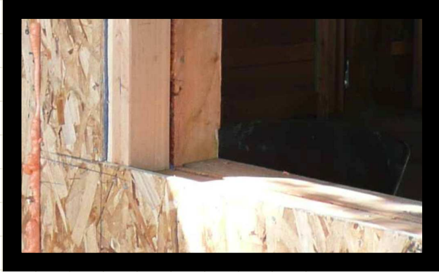
Figure 8. Retrofit Panel Routed for Window Box Courtesy Zero-EnergyPlans.com
