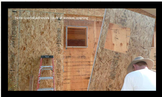
Figure 9. Window Box with Retrofit Panel Courtesy Zero-EnergyPlans.com
