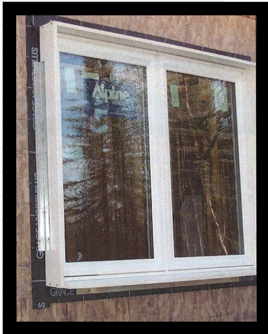
Figure 12. Alternate Window Box Mount Courtesy: Cold Climate Housing Research Center
