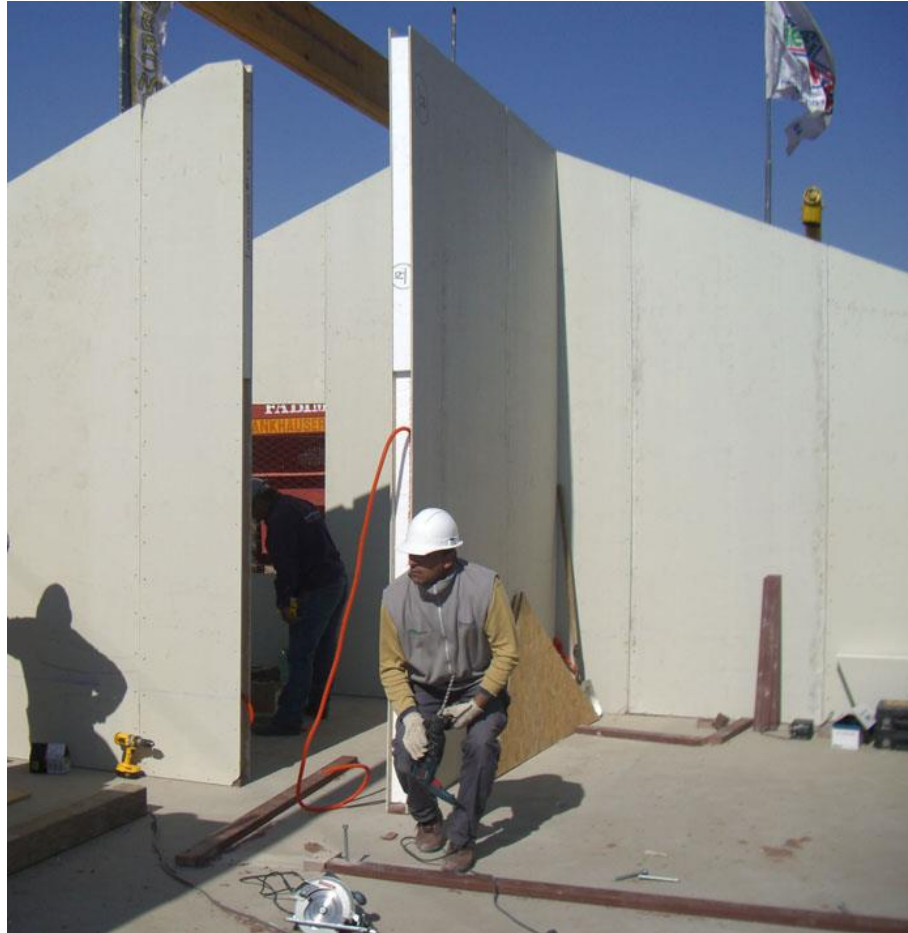
Floor Plate Installation
