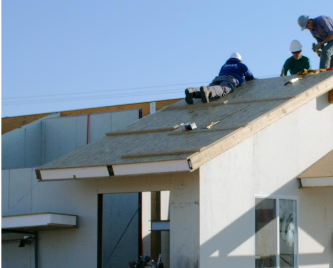
Roof Panel Installation
