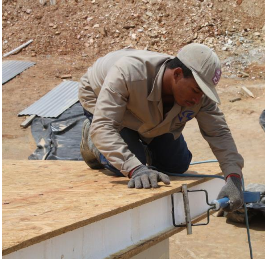
Hot Iron to Clean SIP Sub-fascia
