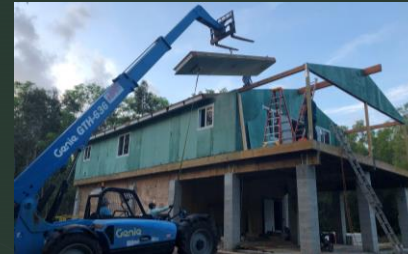
Assembly of Innova Panel Structure
